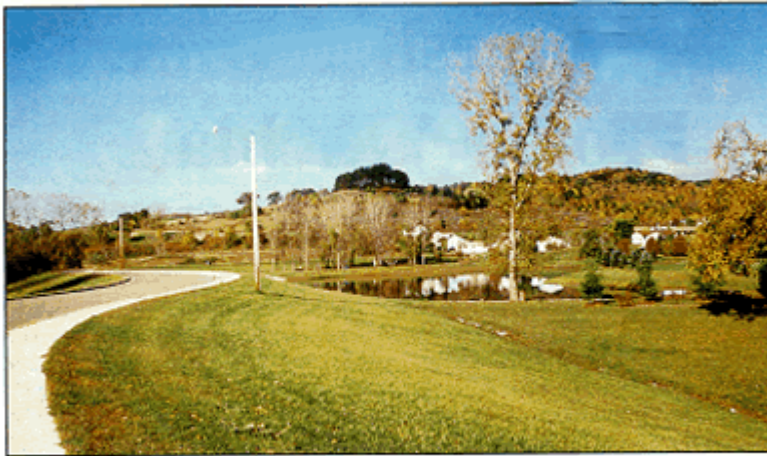
Dike around Allison Park in section where a road was constructed on top. Excavated pond (in center) was stocked with fish and is heavily used, especially by kids.
